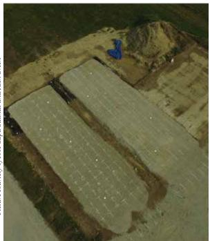
In summer 2020, a team of graduate and undergraduate students assisted in the construction of two testing strips at the Purdue Center for Aging Infrastructure (CAI) Steel Bridge Research, Inspection, Training and Engineering (S-BRITE) Center. The project, aimed at developing guidelines for control of the properties of aggregate drainage layers used in pavement structures, is funded by the Indiana Department of Transportation (INDOT).
